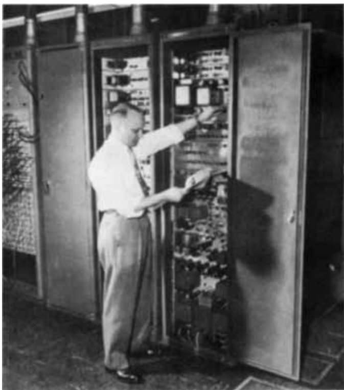
Phonevision's aircode system uses the picture coder, above, to scramble the video portion of the TV signal. Any desired scrambled pattern can be achieved by manual or remote control setting.
