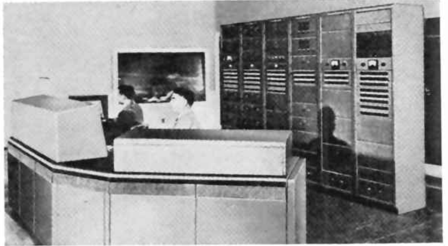
Entire populace can be warned from central control station which can broadcast both alert signals and verbal instructions during and after an attack
