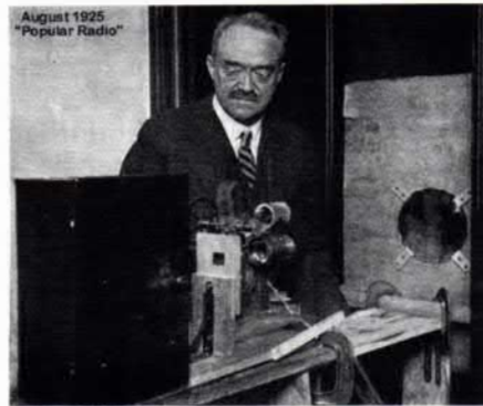
August 1925 "Popular Radio" THE FIRST MOTION PICTURE MACHINE This machine—created by its inventor, C. F. Jenkins—was standard motion picture film. The changing pictures on the film are focused on the flat surface of the lens. The lens which projects these pictures onto the larger lens in the lower end of the two small cylinders directly in front of the inventor.
